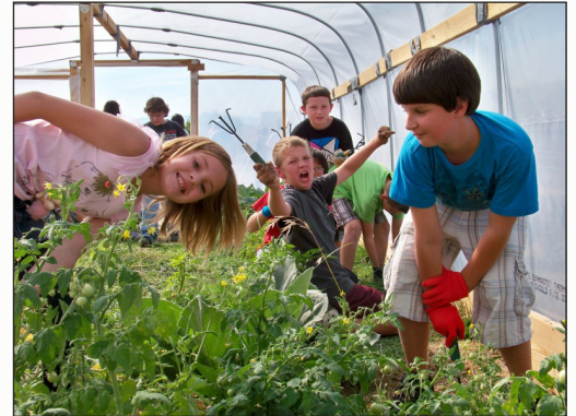
Healthy Communities Coalition—with funding from USDA and the Nevada Health Division and the volunteer labor of parents, students and others—constructed hoop houses at several schools and community gardens in Nevada. Photo by Wendy Madson of Healthy Communities Coalition of Lyon and Storey.
